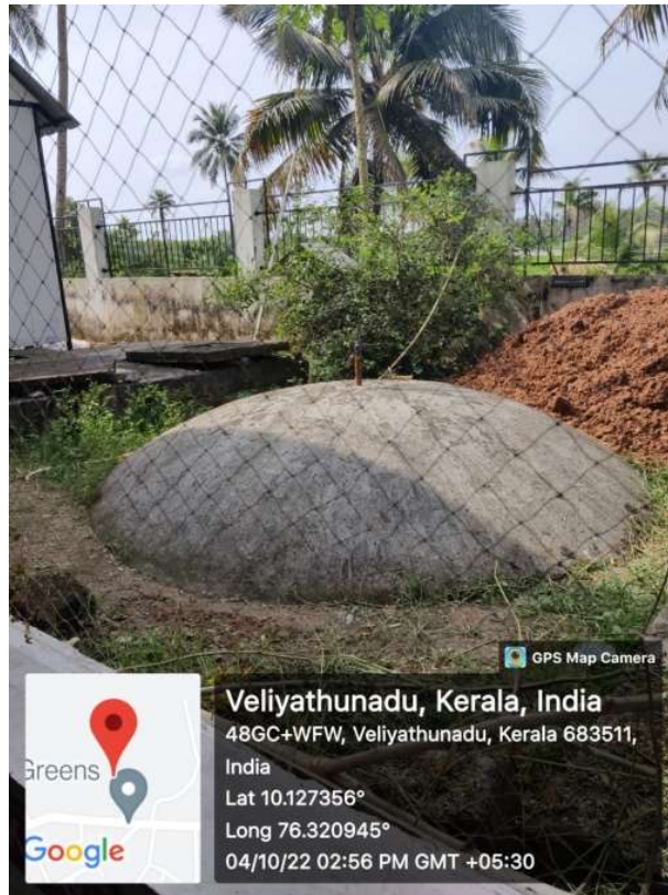
Bio Gas plant
